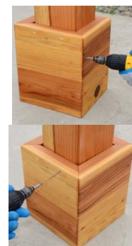
STEP 5: Place the wood boots over the anchors, fixed it with the screws.
