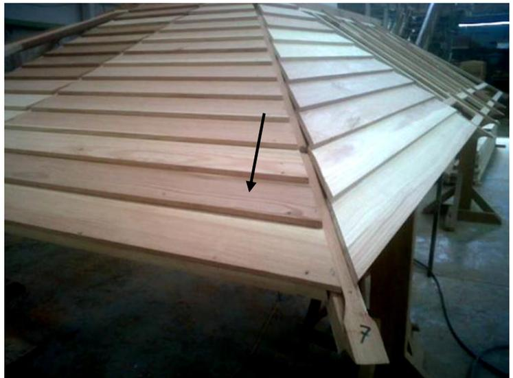
**Step 5:** Attach the roof trim between each roof panel with three deck screws (3" x #8) and repeat the process for each space between the installed roof panels.
