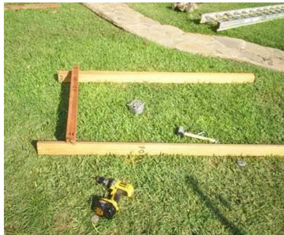
**Photo 3:** Start by building the main wall, this is the door frame of the gazebo.
