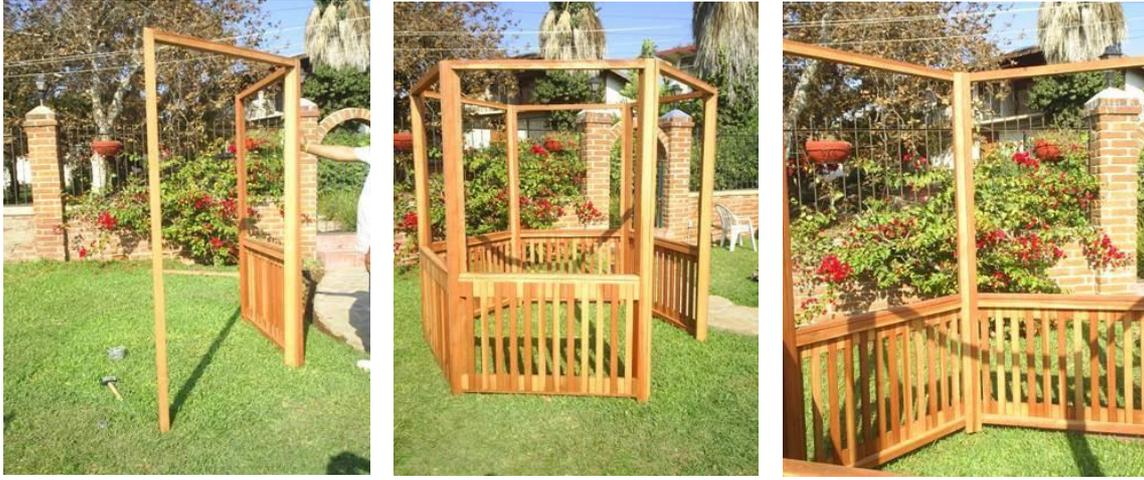
**Photos 5, 6, 7:** Photos 5, 6 and 7 show the door frame completely built, the first wall is set and then the rest finished with all the panels, each joint has 3 bolts.
