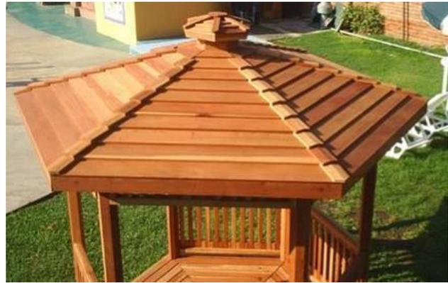
**Photos 11, 12:** Picture 11 shows how each section of the roof is being assembled with two bolts, side to side. On the top there will be a crown that will also help to hold the upper part of the roof, as shown in picture 12. The roof can be fully assembled before is set on top, or installed section by section until it is completed.
