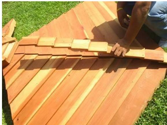
**Photos 13, 14:** To complete the roof, long strips with triangular ends are set with screws on the joints of the roof, as picture 13 and 14 show.
